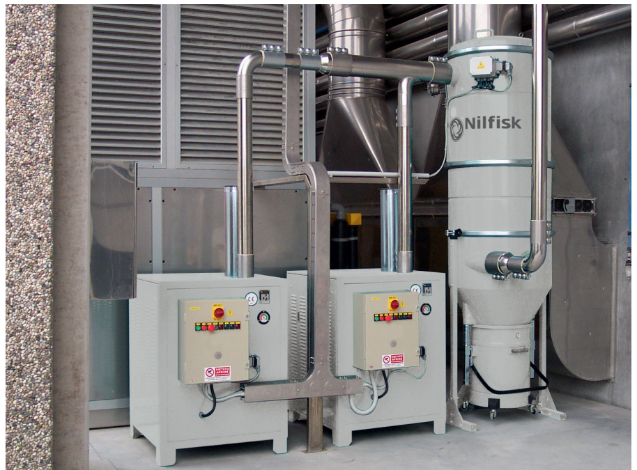
Centralised vacuum system in a chemical company: 2 vacuum units, 1 filter silo.
