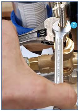
STEP 3 – Tighten counter nut (7)
